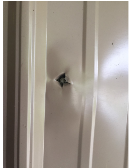
Steel siding blew past screw in pole barn 100 yards from strike.
